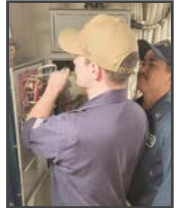
Above: A burnt VR1 relay on an Automatic Bus Transfer (ABT) from USS Ashland was discovered after troubleshooting. Right: EM2 Michael Ingle and EM2(SW) Nestor Caslatan conducting repair on a burnt ABT VR1 relay. (Photos by Rizalito Antonio.)
