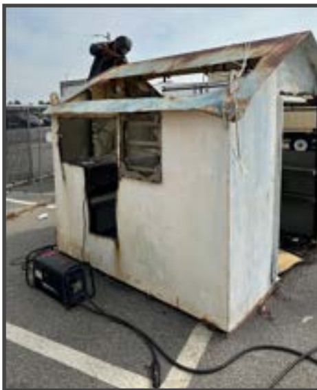
HT3 Austin Dias dismantling a shed on Pier 4 utilizing a plasma cutter. (Photo by HT2(SW/AW) Derek Buss.)
