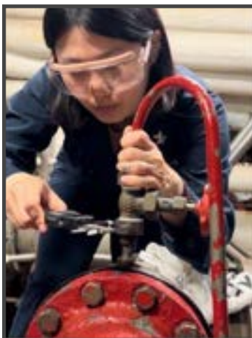
MR2 Wenhui Li takes measurements to verify the correct size of the valve. (Photo by Victor Elias.)
